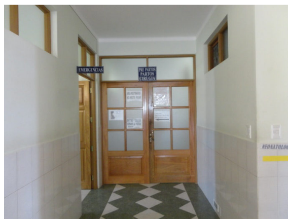
Quirófano de obstetricia, Hospital "San Pedro Claver"
